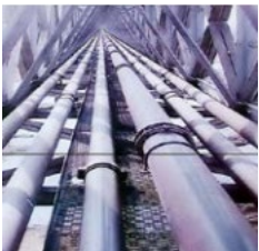
Thickness check of pressure pipelines
