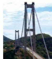
Routine maintenance of roads and bridges
