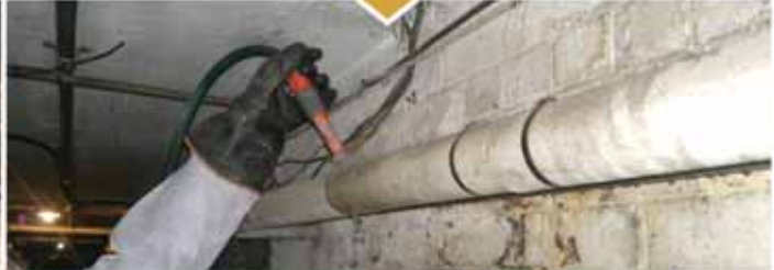
Asbestos Removal & Encapsulation
