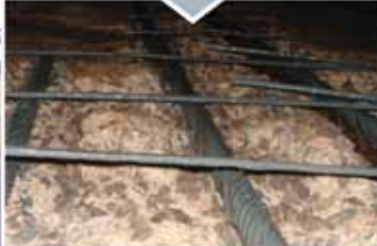
Concrete & Spalling Repair
