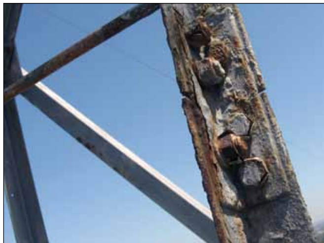
A splice joint in a ladder run is shown, demonstrating how lighter members and where pockets and unsealed connections are more vulnerable. The tower is about 35 years old and was painted with epoxy high build about 13 years ago. Rather than attempt to site clean, prepare and paint these surfaces, it would be better to remove, blast and regalvanise the ladder, make new splice plates and fit these together with new bolts.
