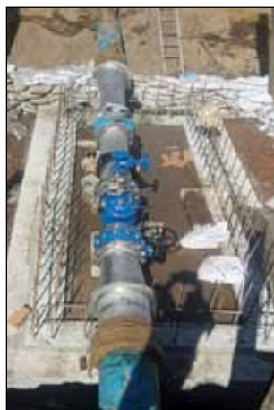
300mm diameter bulk water connection installation for Pearl Valley, Paarl.
