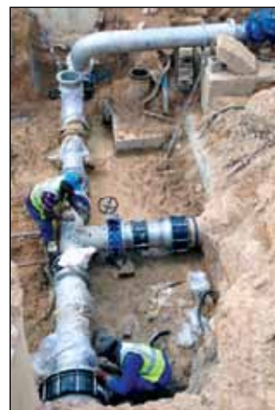
Refurbishment of pipe work at Van Blerk Reservoir, Wellington.
