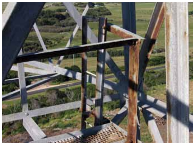
These landing handrails are currently still functional but will progressively lose section thickness and integrity. Therefore, they are not worth spending any time and money on before they are corroded enough to require replacement. However, the main leg members and the compression struts for the cross arms in the background should be cleaned and repainted shortly before their condition deteriorates to the point that the surface preparation intensity rises too far.
