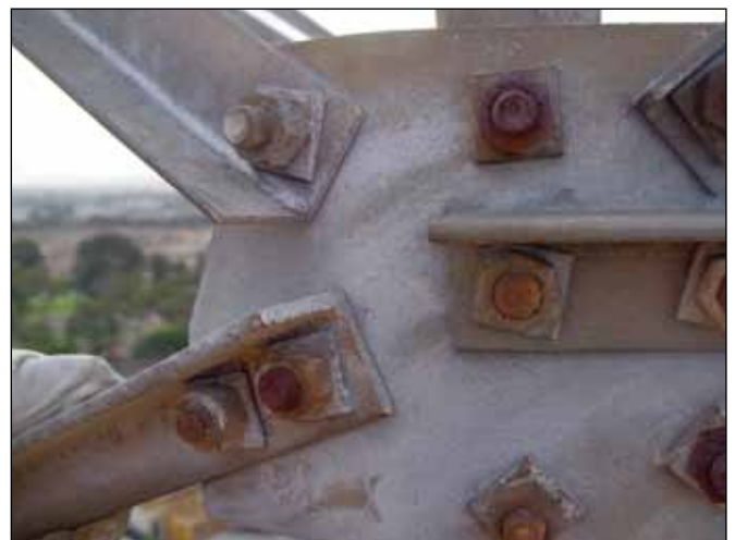
One of the first signs of the loss of galvanic capability is the commencement of gingering of bolts and fasteners. This is partly due to the lower initial thickness of the galvanizing, as such items are usually centrifuged just after withdrawal from the galvanizing kettle. Note the comparative degree of condition of the cleat plate and the affixed angle members versus the bolts.
