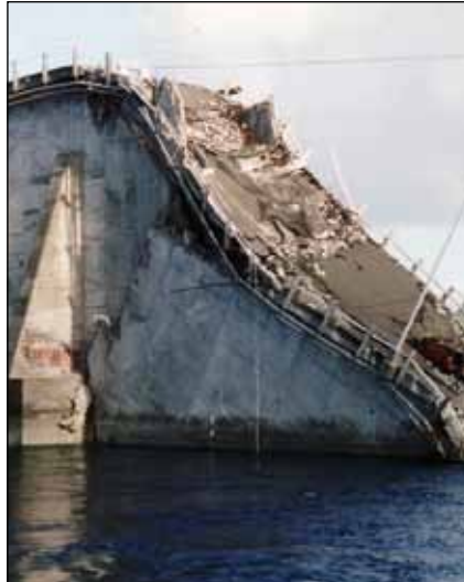
Bridge collapse due to corrosion of steel in concrete.
