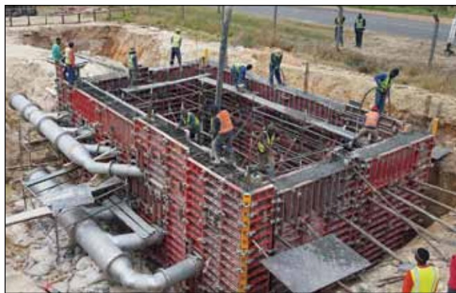
Leliefontein booster pump station.
