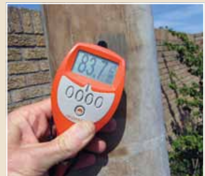
Coating thickness of 83.7µm on the Fe/Zn discolored portion.
