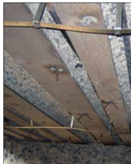
Underslab grid of mixed metal oxide (MMO) coated anode strips installed to significantly retard the corrosion of the underside in situ reinforcement of this concrete slab.
