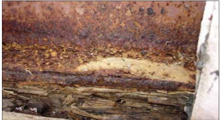
Rusting steel has exposed structural timber which has begun to rot.
