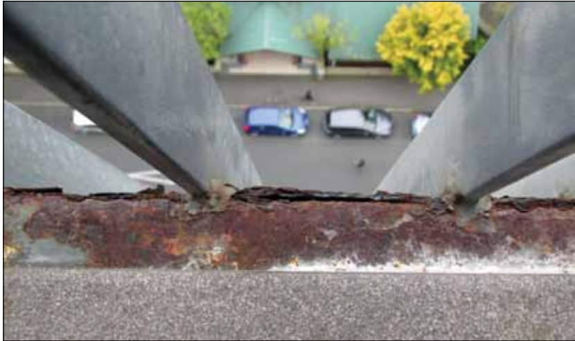
Working 20 storeys above the ground adds to the challenges of protecting structures from corrosion.
