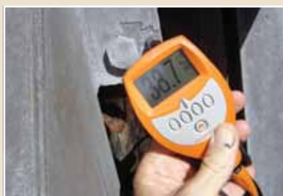
Residual coating of 38,7µm of Fe/Zn alloy layer remains.
