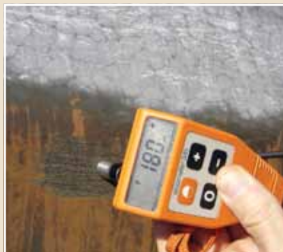
Coating thickness of 180µm on the Fe/Zn discolored portion.
