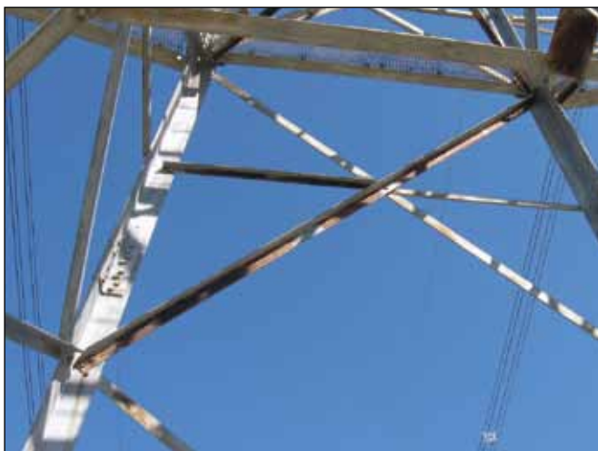
This shows quite dramatically how lighter members and those that have sheltered surfaces not subject to fresh water rain washing, lose zinc thickness and corrode way quicker than heavier and near-vertical members. Replacement of the face braces is not yet due but is relatively easy when required as only a few bolts need to be removed to change out these simple steel sections.
