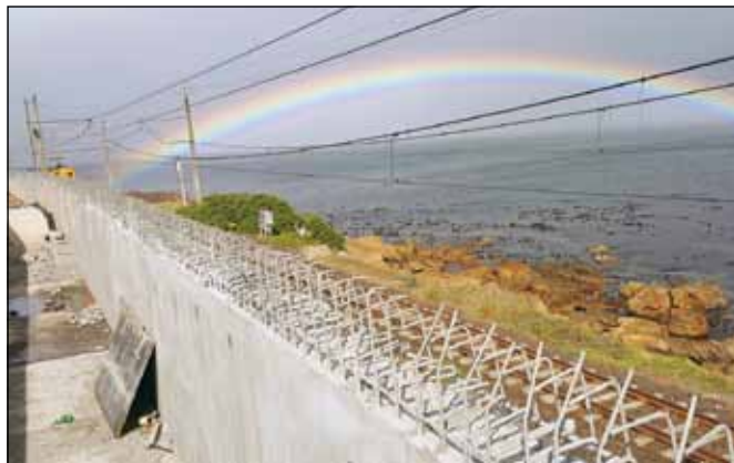
View with a rainbow and a train approaching of the hot dip galvanized high yield starter steel bars for the crash impact designed coping barrier of the Clovelly (Cape Town), retaining wall.
