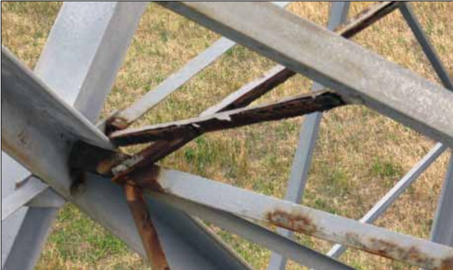
This print shows a good example of how the lighter members, which start with an initially lower thickness of galvanizing, corrode way earlier than heavier members like the main legs. The orientation of the sections also changes the amount and rate of zinc loss. These lighter members are due to be replaced, as attempting to economically and reliably clean and paint these in situ will be futile. The legs members, however, are in a near perfect condition to be cleaned and painted whilst some galvanic capability remains.
