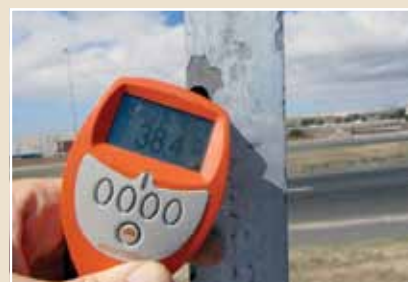
Residual coating of 38,4µm of Fe/Zn alloy layer remains.
