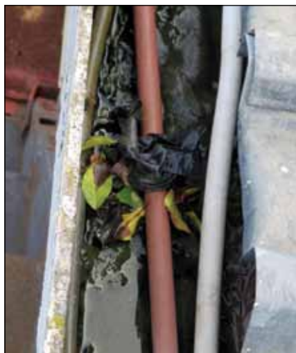
Rain water gutters must be frequently cleaned of all debris and other service pipes should not be laid within them, in order to maintain their integrity.
