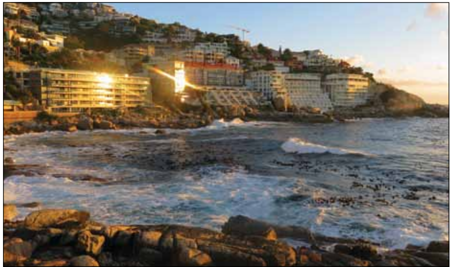
Concrete corrosion can occur rapidly on buildings subjected to marine environments.
