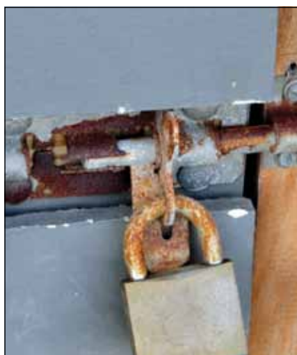
Making use of an inappropriately coated door latch and lock in an aggressive marine environment, will generally result in premature replacement.
