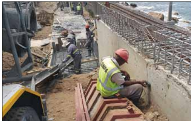
A cover meter was used to check the concrete cover over the hot dip galvanized high yield reinforcing steel, before assembling the steel coping shutters.
