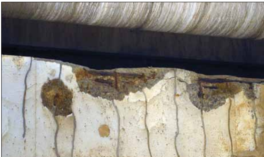
Surface discoloration and cracking of the concrete will ultimately lead to concrete spalling and potential failure.
