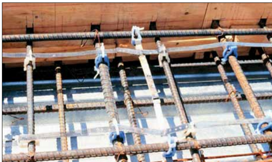
Where de-icing salts have led to the corrosion of the upper reinforcement in this bridge deck, a grid of mixed metal oxide (MMO) coated anode strips have been installed. These will be fully encapsulated with a dense concrete over layer.
