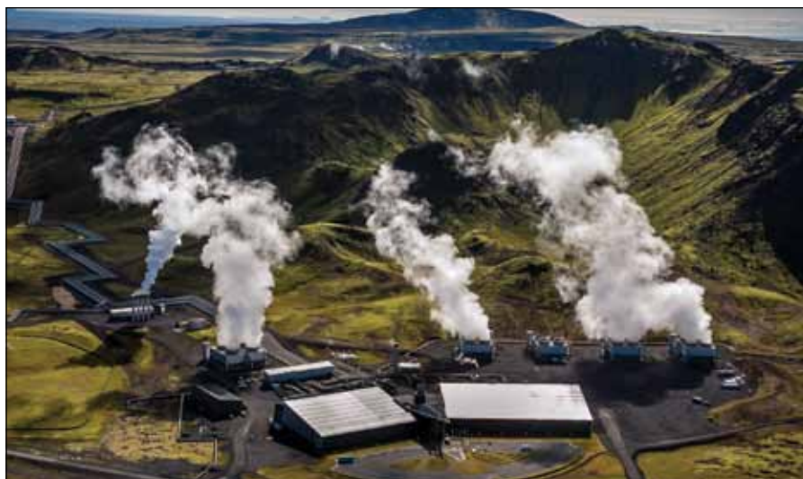
The Hellisheiði geothermal power plant in southwest Iceland. Photo by Arni Saeberg, courtesy of Orkuveita Reykjavíkur (Reykjavík Energy).
