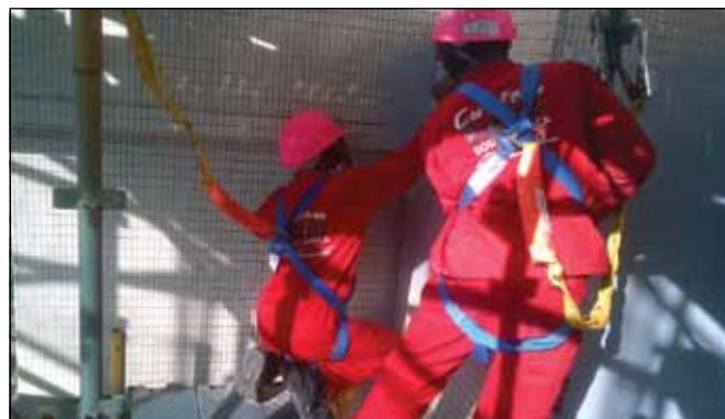
Workers in correct safety equipment preparing substrate for primer.
