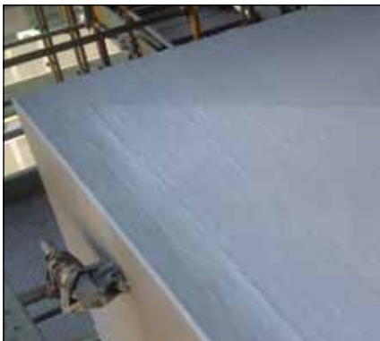
Window sills after application of Ultraspray 401 Polyurea.
