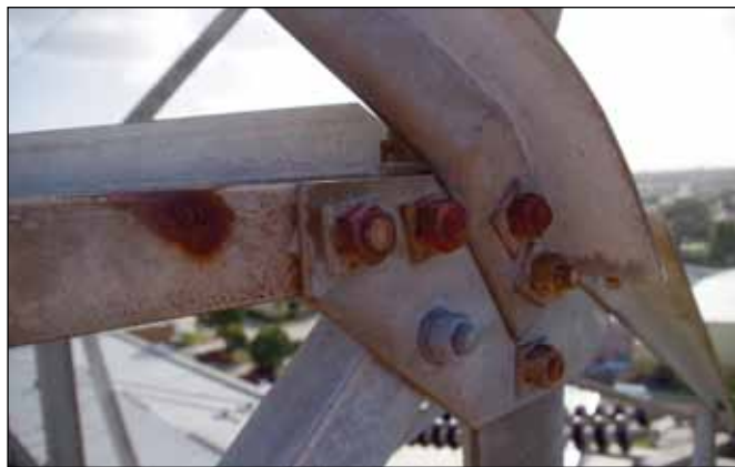
For a galvanized lattice tower located in an urban environment after about 50 years of exposure, this condition would be considered quite typical. However, all members and bolts are still functional, even with some ginging commencing. If the next action is to prepare and paint, then work should be planned to occur relatively soon; however, if replacement like-for-like is adopted, some further life is readily achievable.
