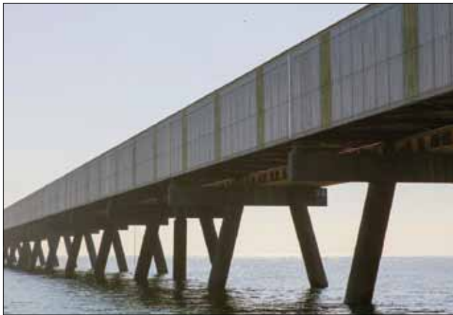
Offshore loading conveyor at Lucinda Bulk Sugar Terminal.
