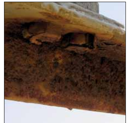
These bolts are more corroded but are actually also still functional, as is the angle brace. Within the next three to four years it would be opportune to replace both the member affected by corrosion and the accompanying bolts.
