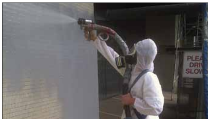
NUI Ultraspray 401 Polyurea being sprayed with a Graco Reactor EXP 2 and a Graco Fusion gun.
