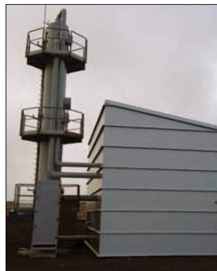
The gas separation system with the absorption tower. Photo courtesy of Sigrún Nanna Karlsdóttir.
