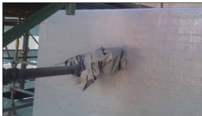
Newly applied Ultraspray 401 Polyurea.
