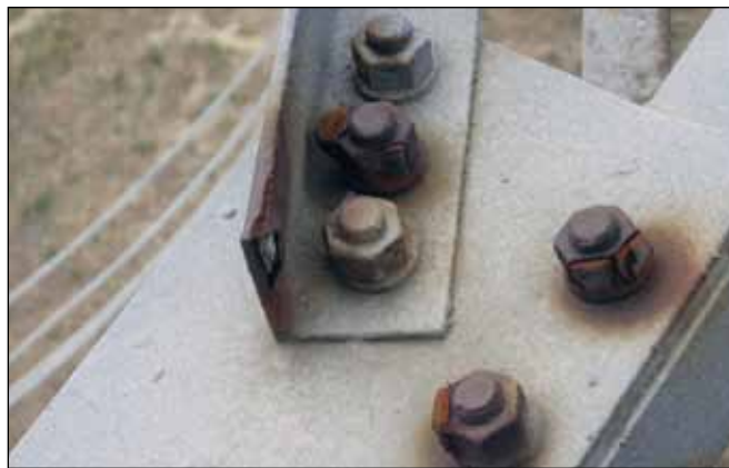
These are good examples of corroding bolts. However, these are nowhere near in need of replacement as their functionality is not yet in doubt. These have been painted in the past but it is not recommended that any effort should be expended on cleaning and painting these as it would be a poor reward for the effort expended.
