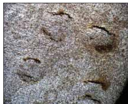
An image of the surface of the S235JR CS specimen after four weeks of testing, taken with an optical microscope equipped with a digital camera. Large cracks and blisters are clearly visible. Photo courtesy of Sigrún Nanna Karlsdóttir.
