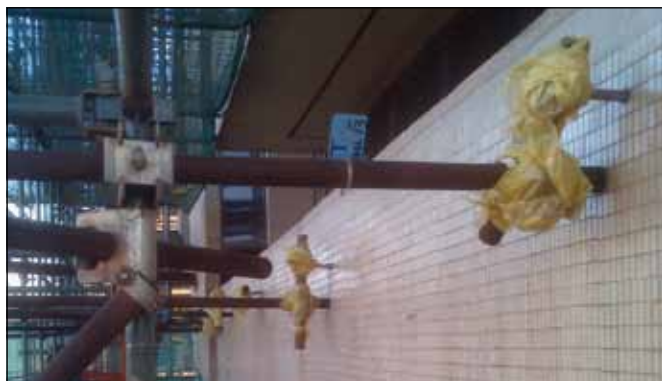
Scaffolding erected against ABSA Towers. Glazed tiles ready to receive NUI formulated glaze tile primer.
