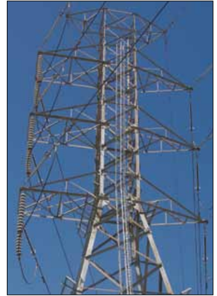
This is a medium strain tower after just over 50 years of exposure. Note the commencement of ginging on the main legs members just above the lower limit of the ladder and around the waist near the lower cross arms. Legs, other primary members and sections in compression should be protected from any advanced corrosion or section loss. It is best to clean, prepare and coat these with a high performance coating system before they lose most of the galvanizing protection.
