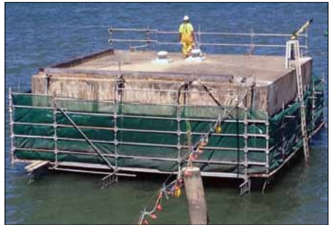
Mooring dolphin at Cairns Bulk Sugar Terminal scaffolded for concrete repair works.
