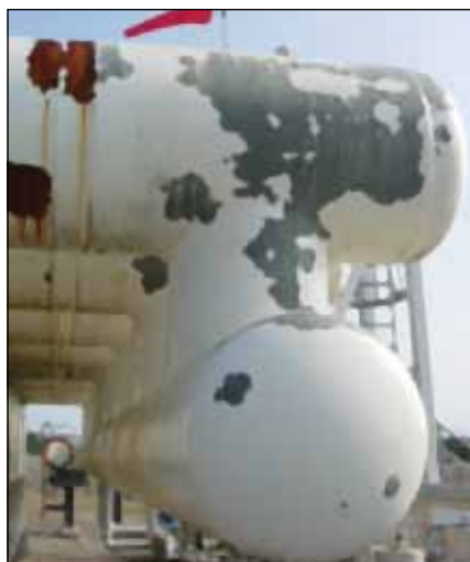
A white, polysiloxane topcoat delaminated adhesively from an organic zinc-rich primer on a pressurized vessel at a gas processing facility. Additionally, the coating system installed in the field-joint area delaminated to the bare steel (as shown in the upper left portion of the picture).
