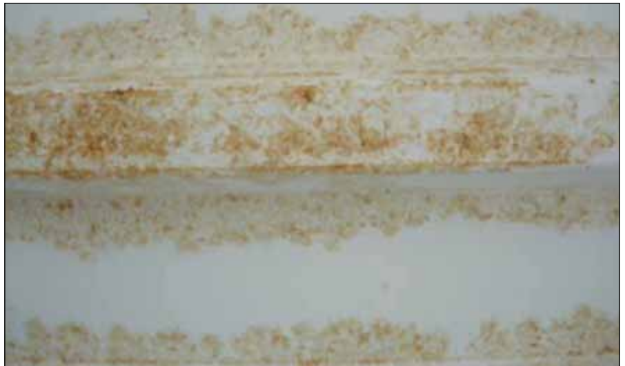
Poor spray application techniques used to apply a coating system on a corrugated interior roof resulted in low dry film thickness in some areas. The structure was open on the windward end and regularly subjected to ocean breezes. The coating deteriorated within six months in areas with insufficient dft.
