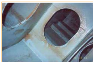
A big improvement with the new coating system
