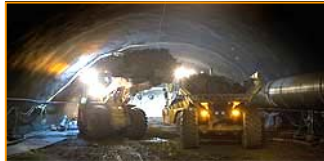
Construction of the Mullum Mullum Tunnel
