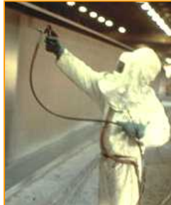
Spraying paint on a steel bridge beam
