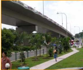
In the past, all the concrete highway flyovers were always left uncoated. The Singapore government have now accepted that the lifespan of each concrete structure can be significantly increased when a protective coating is applied to it.
