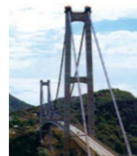
Routine maintenance of roads and bridges
