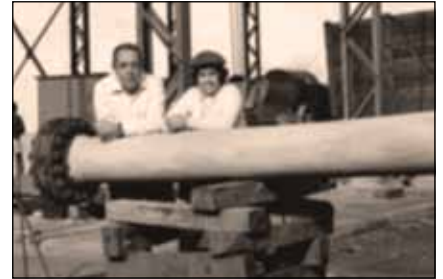
Beira Pump Station under construction.
