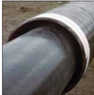
Rehabilitated casings.
