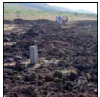
Groundbed markers installed.
