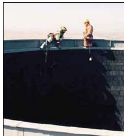
Application at top drain.
