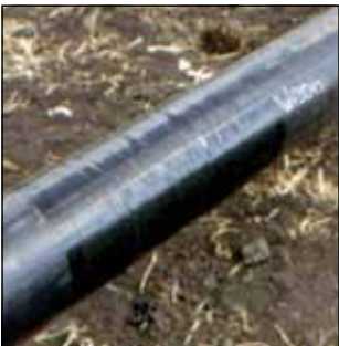
1990's – New factory coated pipe with tape wrap field joints.
