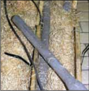
Shattered anodes cause delays.
