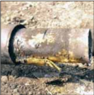
Shorted road casings.
