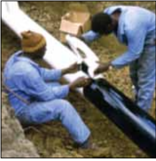
Localised wrapping repairs and CP augmentation.
