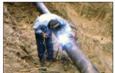
Butter welding on a LIVE pipeline.
