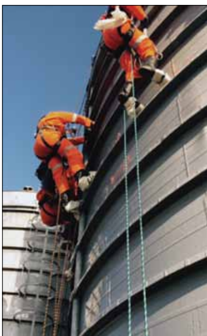
Application via rope access.
