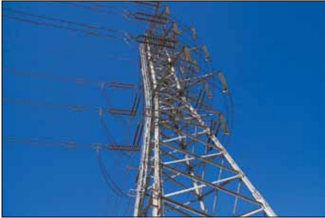
A galvanized lattice strain tower on a 220kV urban transmission line. This structure is heavier than most because it is placed at a corner of the line and is subject to higher side loads, thus the multiple angle members in the main legs and heavier bracing. The regularity of the galvanized steel members and the nature of bolts for assembly are visible.
