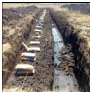
Sectionalised anode installation.
