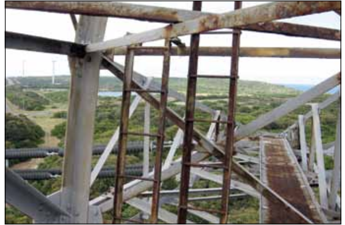
This is the upper cross arm on a 500kV tower located in a near coastal environment. This tower is about 35 years old and was site painted about 13 years ago with a high build epoxy coating system. The extent of corrosion, in spite of the overpainting, particularly of the lighter and partly sheltered members, is readily discernible.
