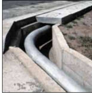
Rerouting the pipe on the new bridge.
