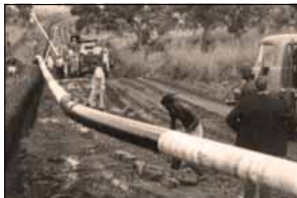
Pipeline construction underway.
