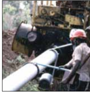
Reclaimed pipe being wrapped.
