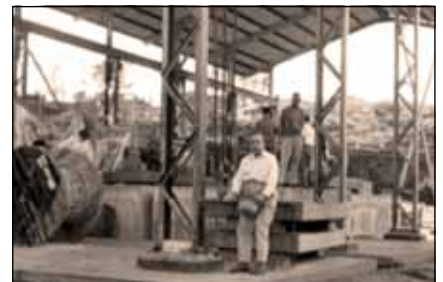
Maforga Pump Station.
