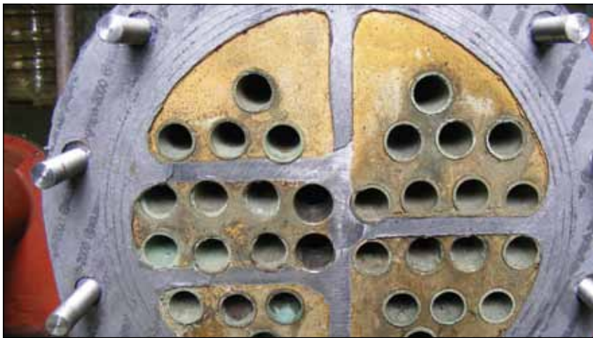
Figure 3: View of the end plate of the failed condenser tubes.
