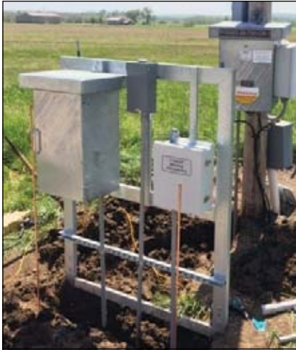
Typical CP rectifier station set-up.
