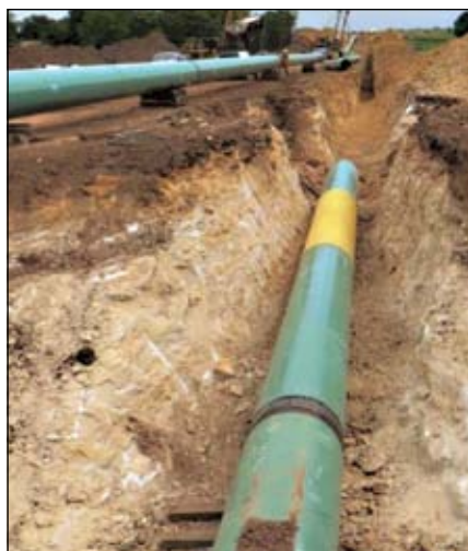
Fusion bonded epoxy coatings are often used on pipelines.
