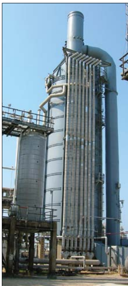
What lurks beneath? Much of the corrosion at a processing plant is rarely obvious.
