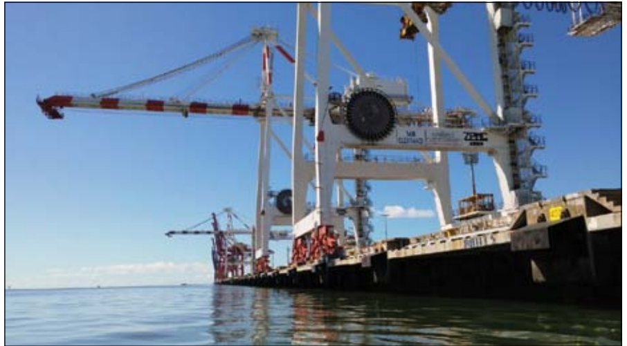
An impressed current cathodic protection system was installed and commissioned in 1999 on Wharves 4 and 5 at the Port of Brisbane in Queensland, Australia.
