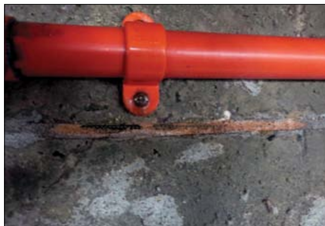
Acidification of the grout encapsulating the ribbon anodes. Photo courtesy of Atef Cheaitani
