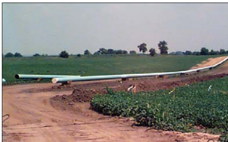
Corrosion protected pipes ready for installation.
