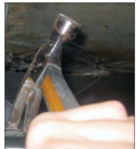
It took a crew of six people, accessing the structure by boat and land, about two weeks to hammer test the entire concrete surface underneath the wharf. Photo courtesy of Atef Cheaitani
