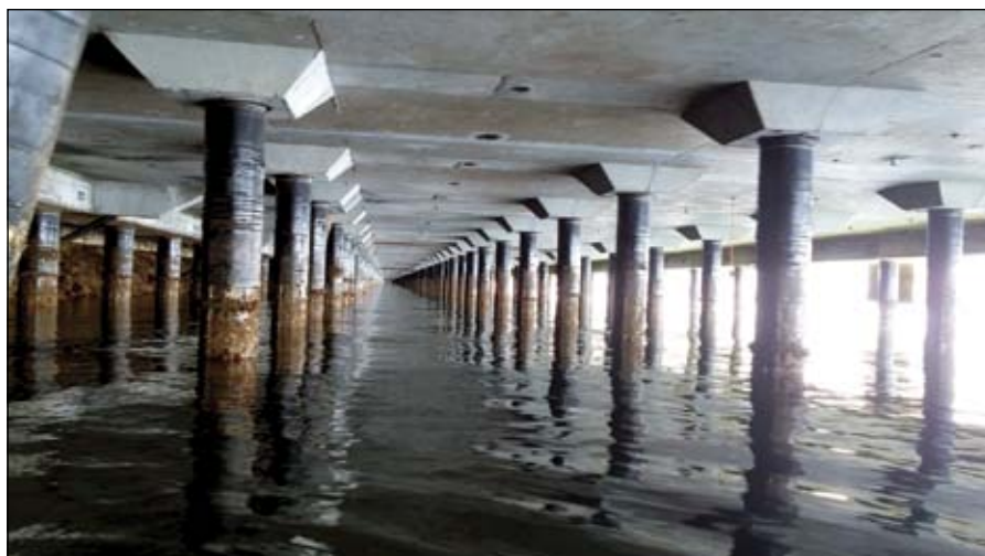
The approximate concrete area underneath Wharves 4 and 5 that is protected by the ICCP system is 8 000m 2 . Photo courtesy of Atef Cheaitani
