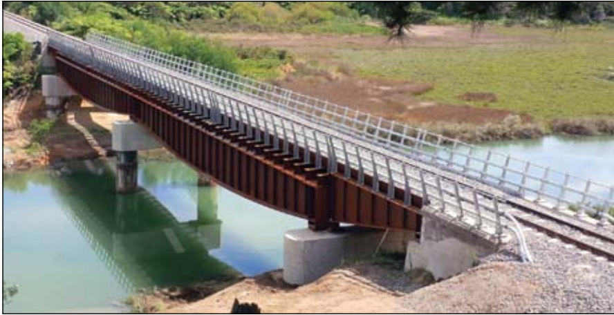
'Weathering steel' narrow-gauge rail bridge in New Zealand.
