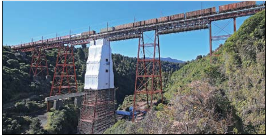
Centre pylon of the Makatote viaduct in New Zealand prepared for restoration. (© 2016, TBS Group)
