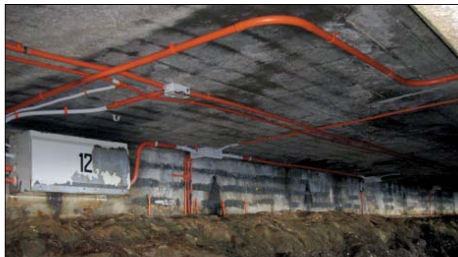
A control unit installed underneath the wharf as part of the original ICCP system. Photo courtesy of Atef Cheaitani
