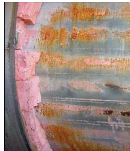
Extensive corrosion discovered under pipe insulation.
