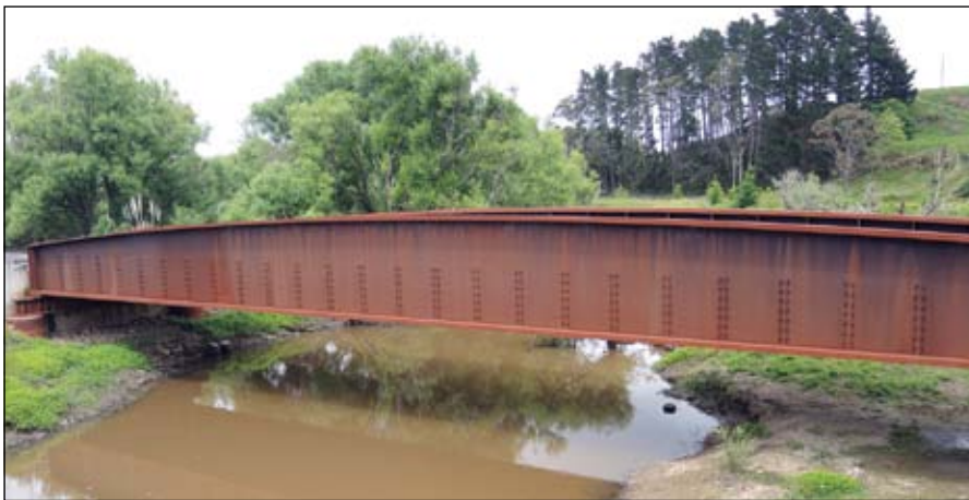
'Weathering steel' girder bridge.
