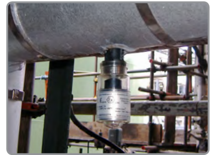
Fitted to the underside of pipelines the Elcometer 1001 collects fluid as it flows to the lowest point
