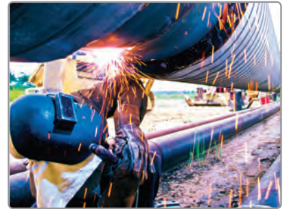
Pipeline failure through corrosion under insulation causes supply shortfalls, economic loss and environmental pollution
