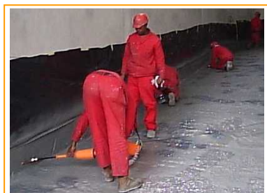
Elcometer 266 with second handgrip and right-angle electrode confirms there are no holes in the waterproof membrane
