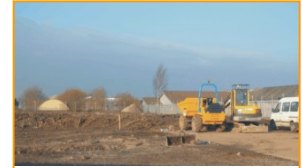
Clearing the way for the 3240m 2 (34875 sq.ft) construction project.
