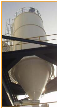
Silo made from vitreous enamelled steel sheets. (Image courtesy of Silo System)
