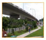
In the past, all the concrete highway flyovers always were uncoated. The Singapore government have now accepted that the lifespan of each concrete structure can be significantly increased when protective coating is applied to it.
